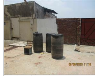
Photo of non-conformity Secondary containment was found missing.jpg
